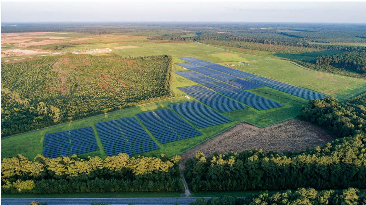
Solarpark „Aulander“ in North Carolina (7 MWp) – Renew Petra
